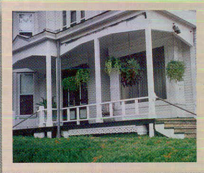
When the Ruppman's purchased the home, its once-grand porch had been replaced with a much simpler design. The Ruppman's decided to return it to its original grandeur.
