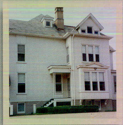
The home's original brackets were removed by previous owners and other ornamental detail was lost under the aluminum siding. The Ruppman's invested heavily in the exterior, re-creating every detail as it once was.
