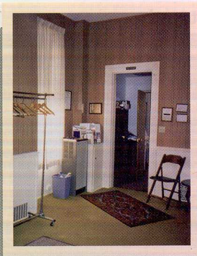
Left: The Ruppman's shifted the doorway in the center of the photo to make room for the refrigerator. They also removed the dated paneling and carpeting, and replaced the light fixture.
