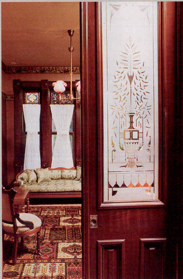
A nice surprise awaited the Ruppman's when they pulled these pocket doors out of the wall: beautiful wheel-cut glass inserts in excellent condition. The doors were formerly blocked in the wall by the carpeting.
